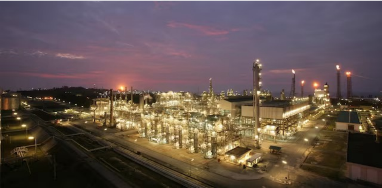
World's first commercial GTL plant, Bintulu, Malaysia.
